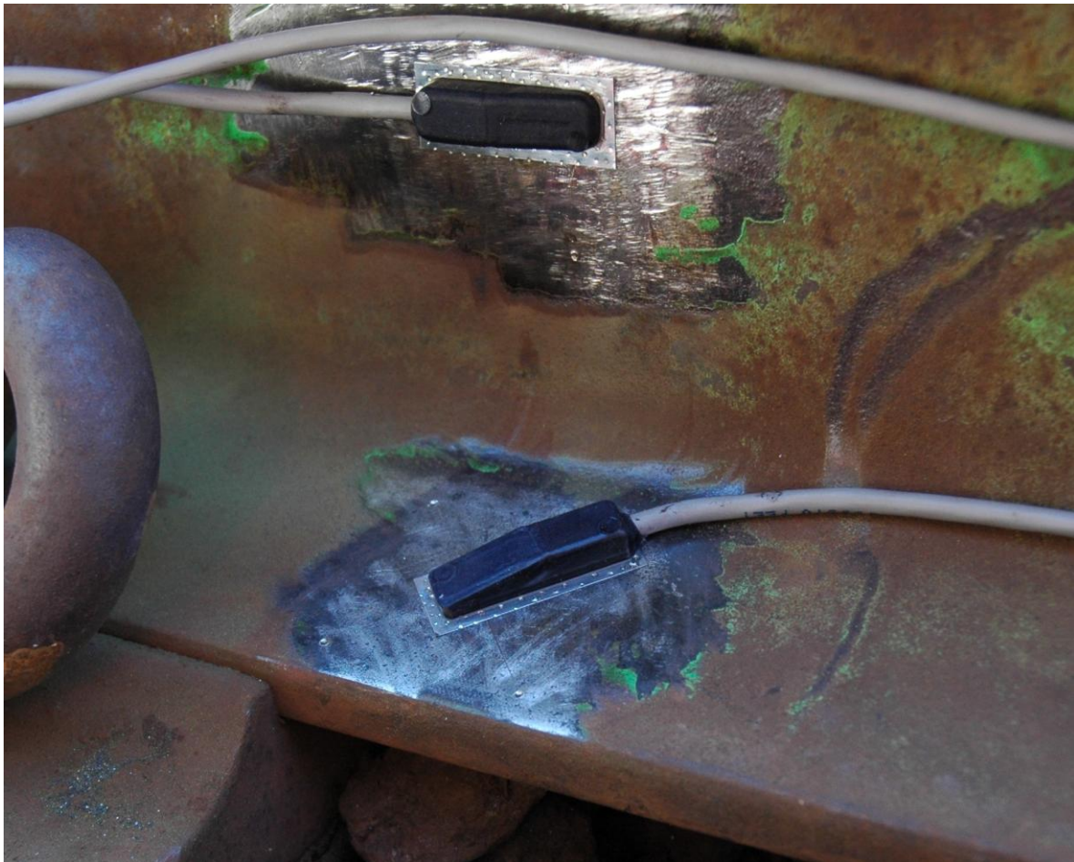
Figure - Strain gauges bonded to rail web and rail base.
